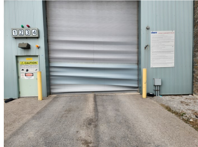
Photo 10: View of damaged Tipping Building east door.
