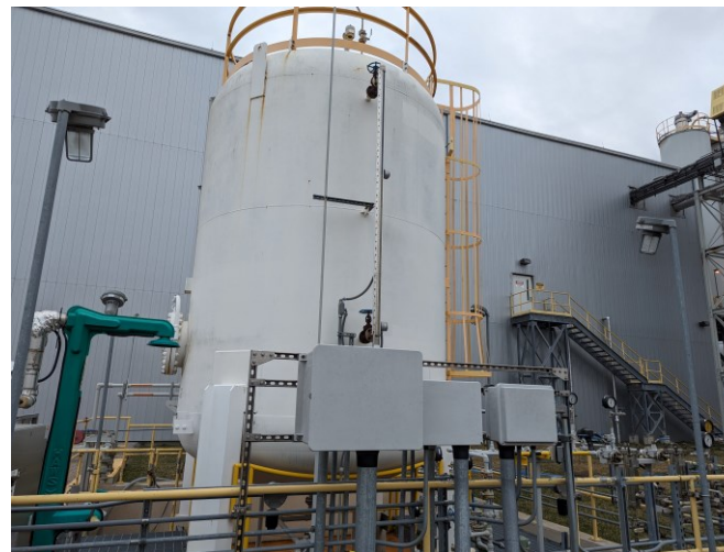
Photo 26: View of the ammonia storage tank.
