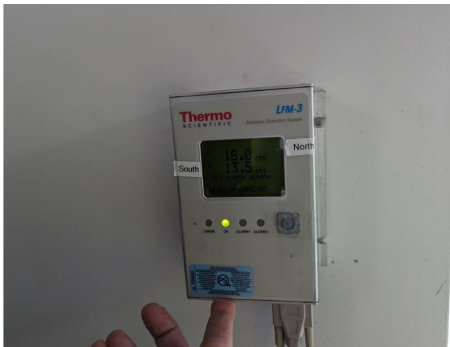
Photo 25: View of radiation alarm in Scale House.
