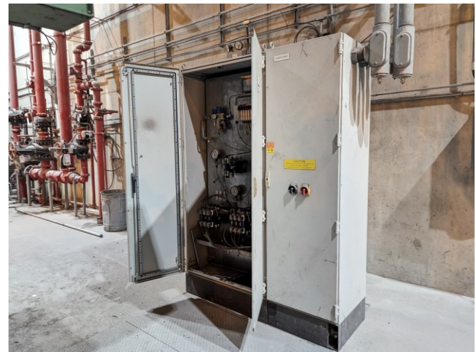
Photo 16: View of open hydro-pneumatic control cabinet in the Boiler Building.
