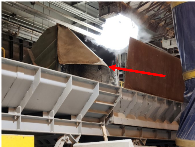
Photo 15: View of damaged ash cover in the Boiler Building.
