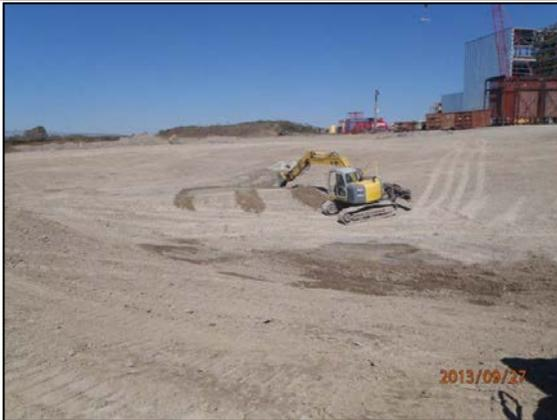
*Photograph 45: View of W-SWMP final grading efforts during dry conditions on September 27, 2013*
