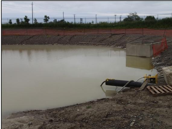
Photograph 25: Closer View of E-SWMP-OUT location showing outlet invert versus water level on June 28, 2013
