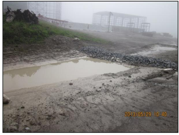
*Photograph 4: Closer view looking southeast/downstream of western swale rock-check dams on May 29, 2013*
