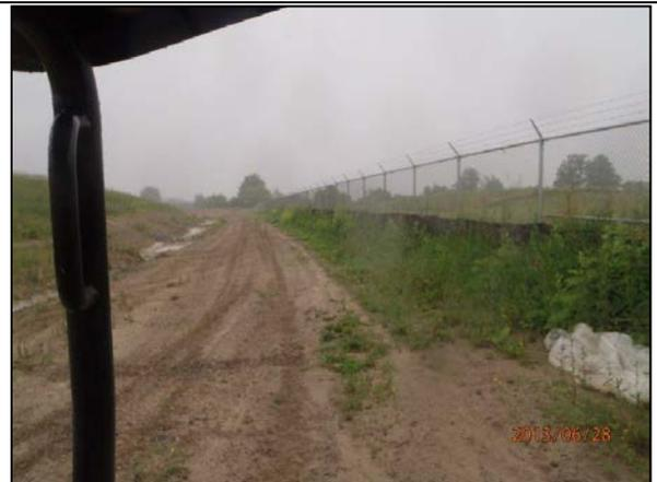
Photograph 22: View looking south capturing western perimeter silt fence and interceptor swale on June 28, 2013
