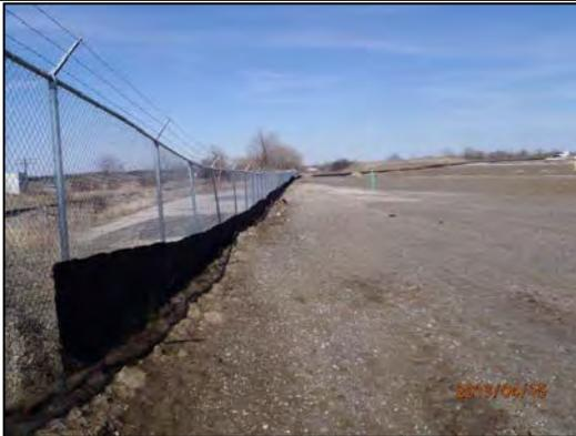
Photograph 69 View of southern perimeter silt fence on April 15, 2013
