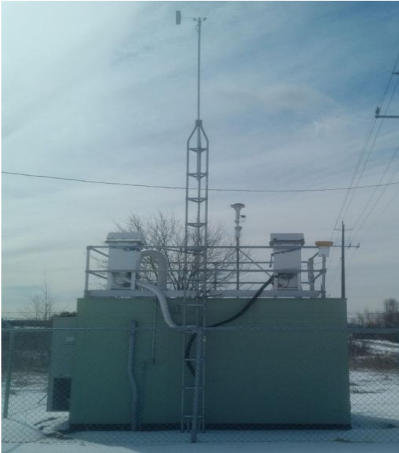
Figure 2: Rundle Road Station
