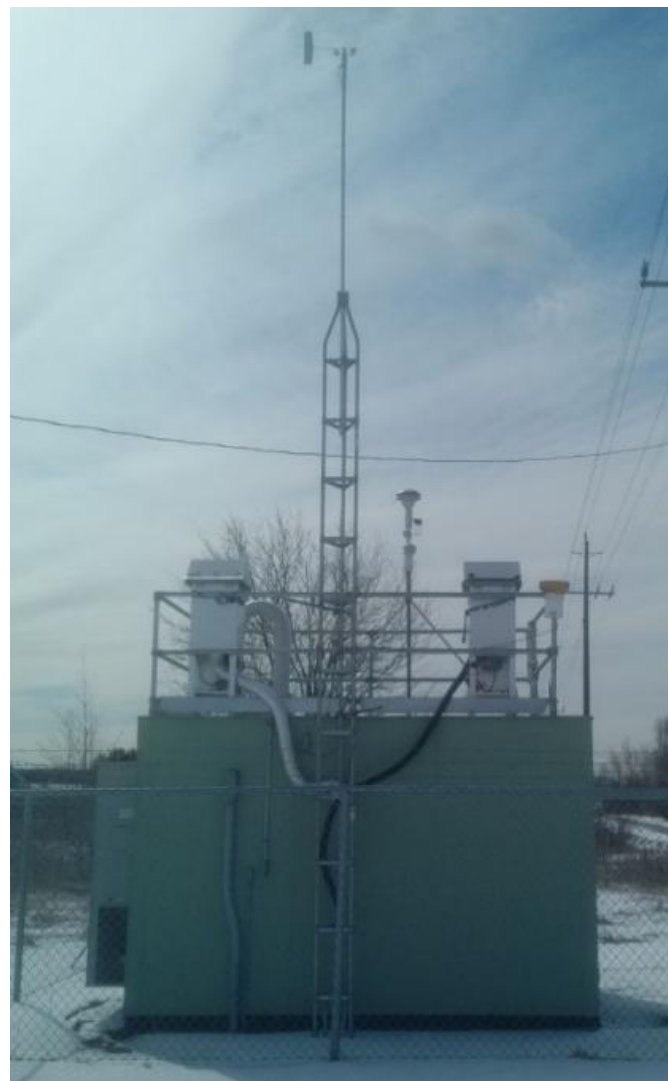
Figure 3: Rundle Road Station
