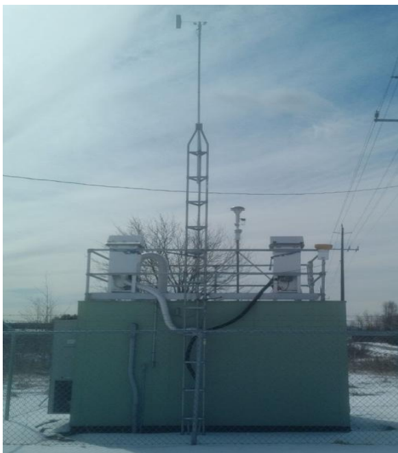
Figure 2: Rundle Road Station
