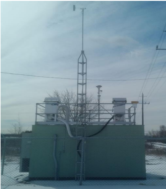
Figure 2: Rundle Road Station
