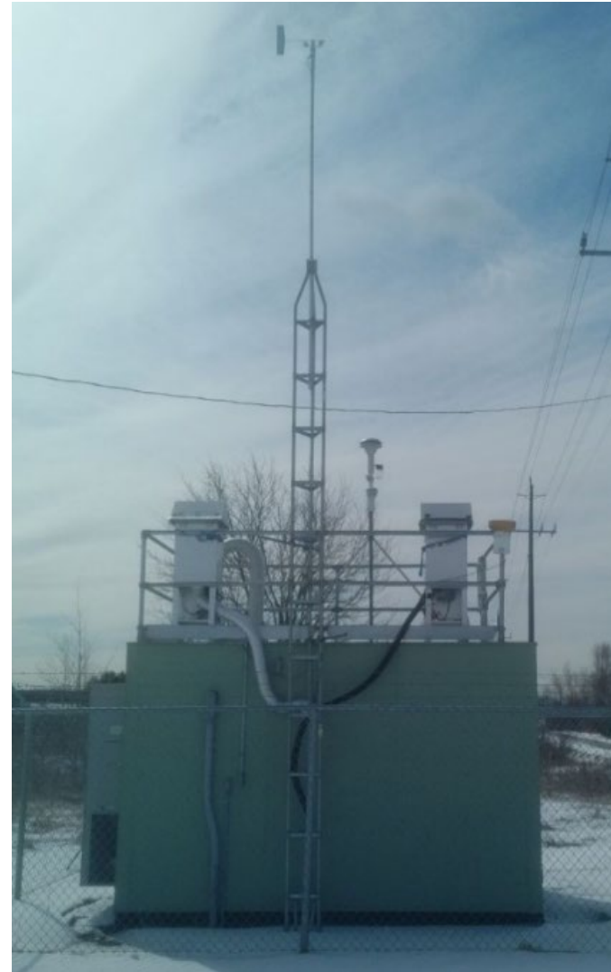
Figure 3: Rundle Road Station
