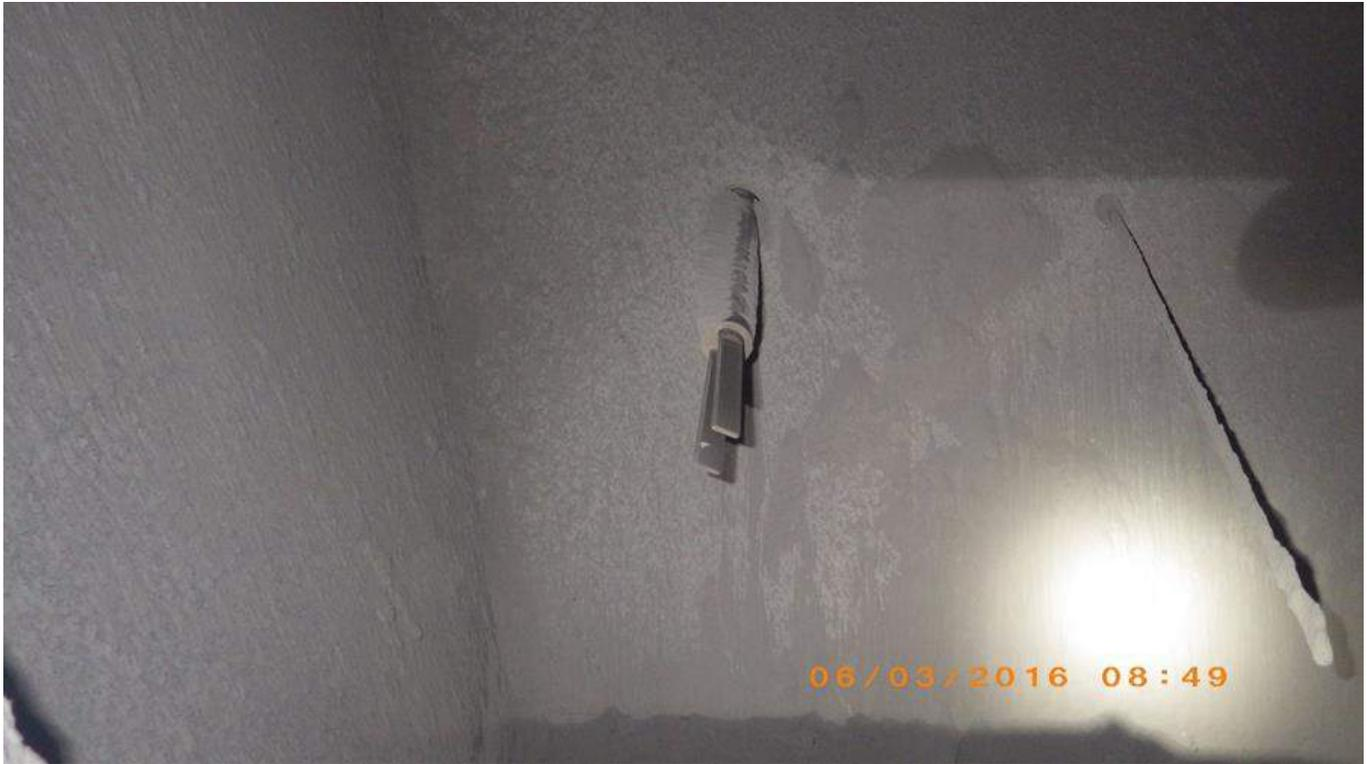
Photo 27 - Baghouse 1 -Hopper Level probe – Installed With Incorrect Orientation (Gap should be vertical)
