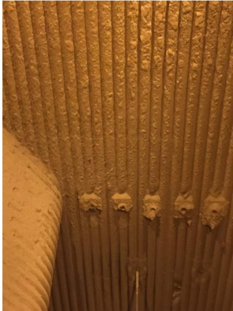
Photo 2 – Boiler 1<sup>st</sup> Pass – IGR Nozzles
