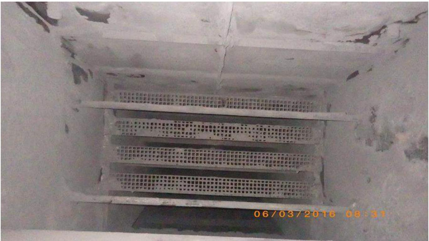
Photo 38 - Inlet To Baghouse Inlet Duct – Baffle Screens at Far End Cleared during Boiler #1 Shutdown (as left)
