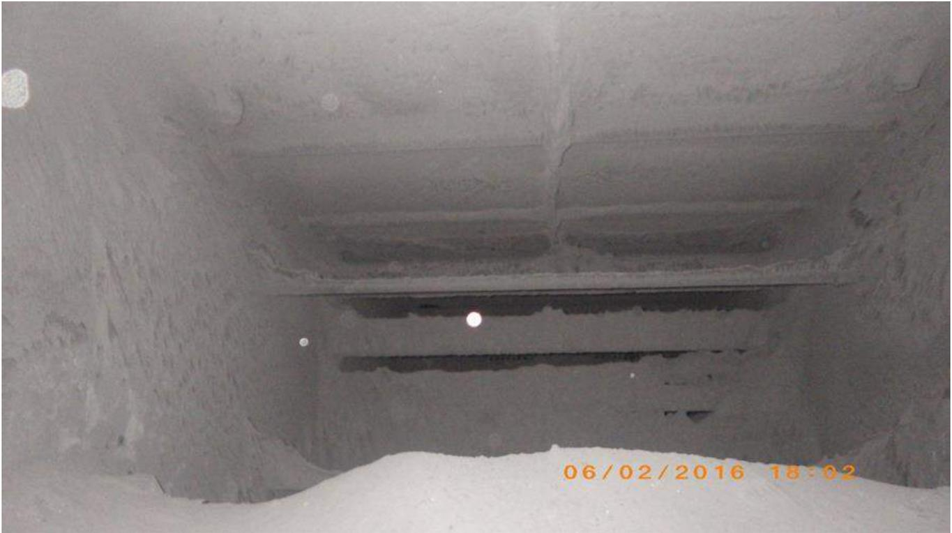
Photo 37 - Inlet To Baghouse Inlet Duct – Baffle Screens at Far End Plugged (as found)
