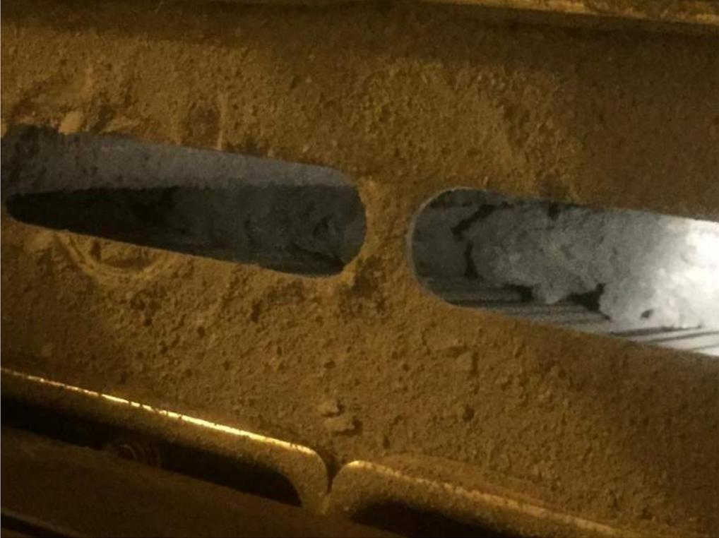
Photo 25 - View of Buildup Between Bags – NOT TYPICAL
