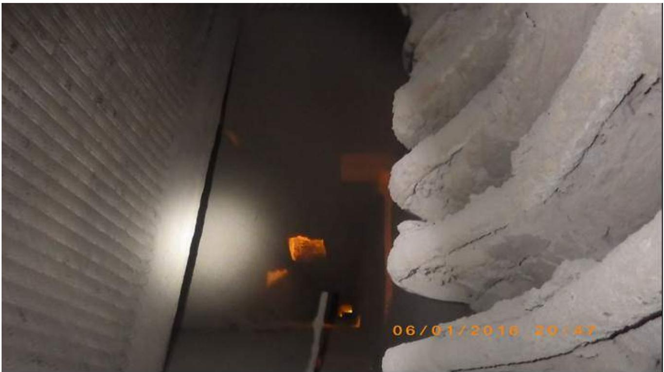
Photo 9 - 3<sup>rd</sup> Pass Rear wall – Loops from Convective Zone Removal on Rear Wall (left side of photo)
