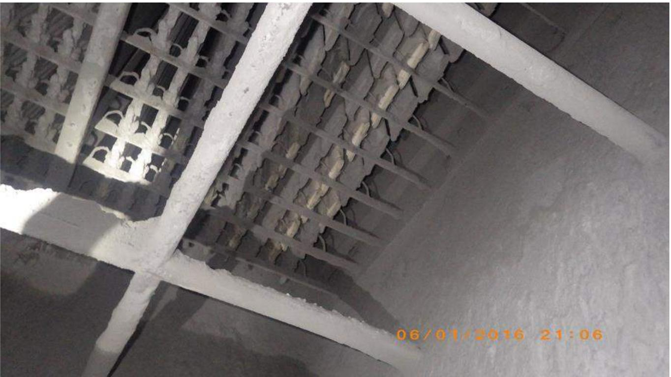
Photo 21 - Bottom of Baghouse Bags – Replaced bags are Evident
