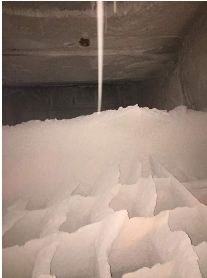
Photo 30 - Vanes at Discharge of Quench Reactor – some Buildup – Not Considered Excessive
