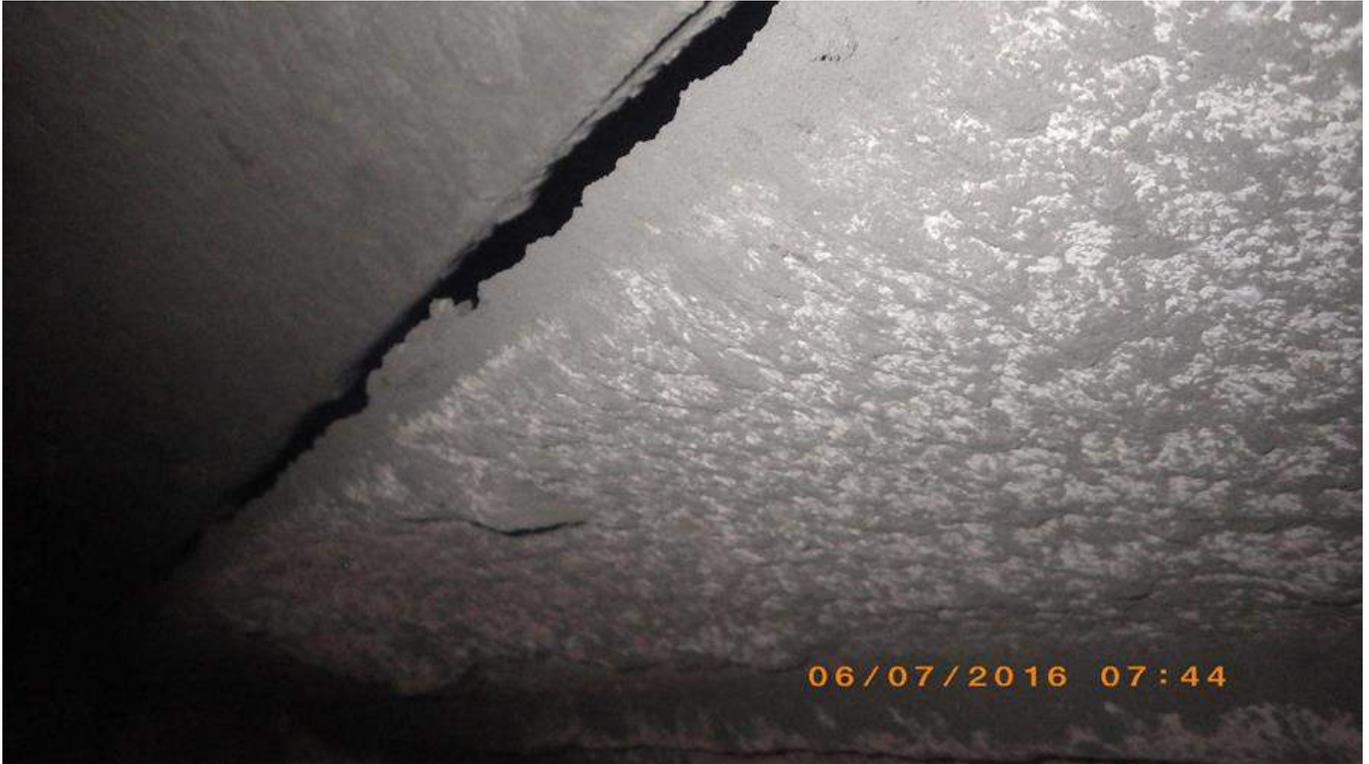
Photo 33 - Damper between Quench and Dry Reactor. Only Slightly Open – Forces air down into Conditioning Rotor
