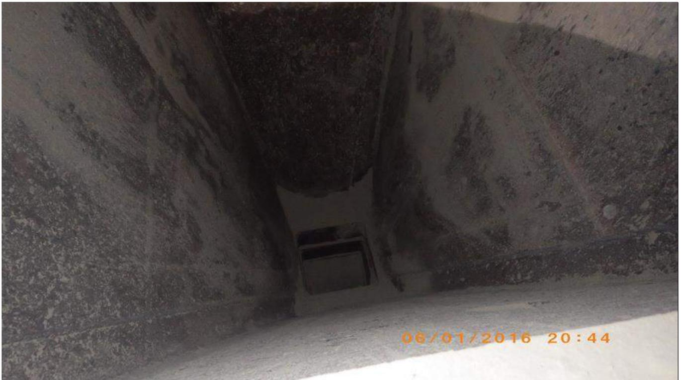
Photo 16 - Hoppers under Superheater Sections - all Clear
