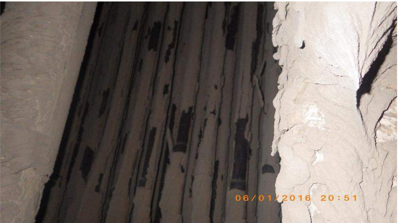
Photo 11 - Upper 3<sup>rd</sup> Pass – View Looking into Superheater – Screen Tube Fouling Heavy Near Door
