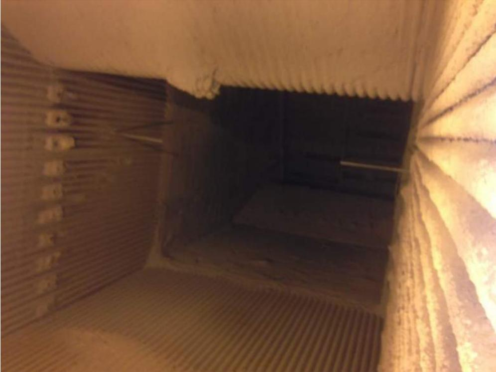
Photo 3 – 1<sup>st</sup> Pass Small Build Up on Bullnose
