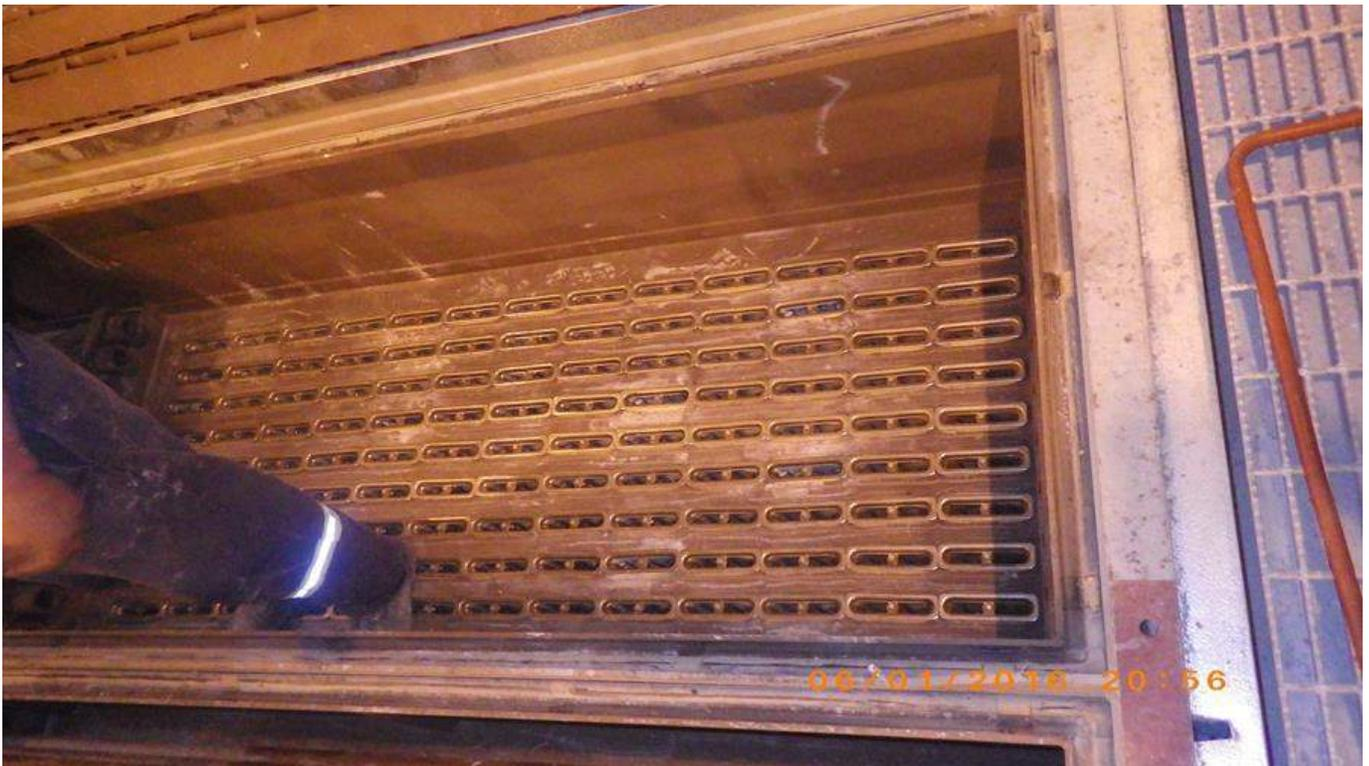
Photo 19 - Baghouse Tube Sheet – Dust Indicates Bags in That Area Have Been Pulled for Replacement or Inspection
