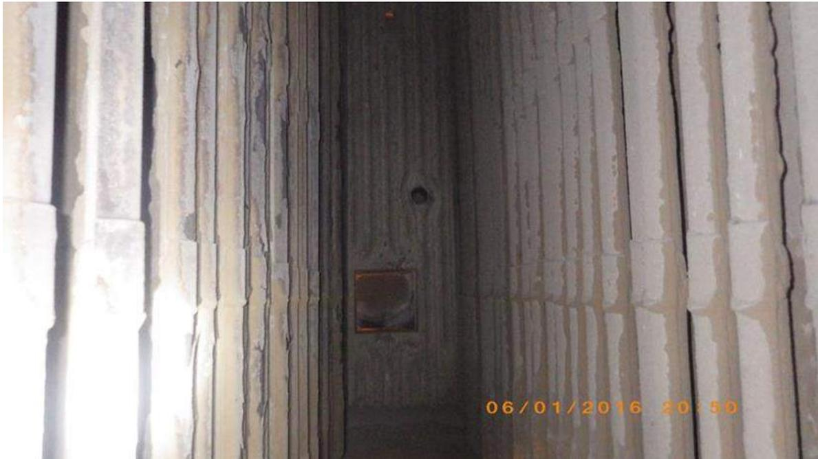
Photo 14 - View Between Superheater Sections – Fouling Typical
