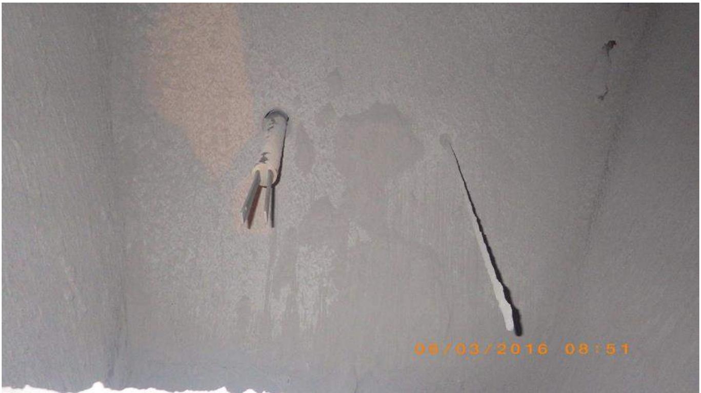
Photo 28 - Baghouse 1 -Hopper Level probe – Installed With Correct Orientation (Gap vertical)
