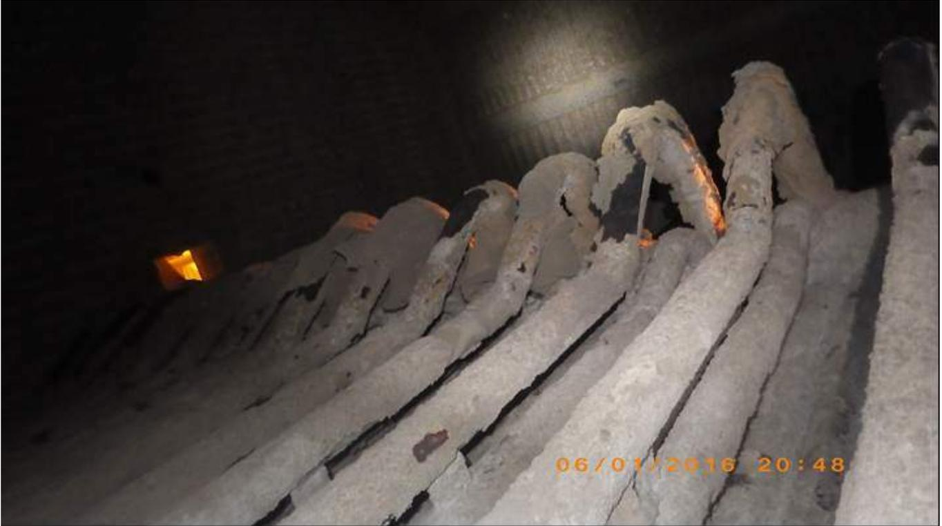
Photo 10 - 3<sup>rd</sup> Pass Convective Zone Bypass Loops – Looking Up
