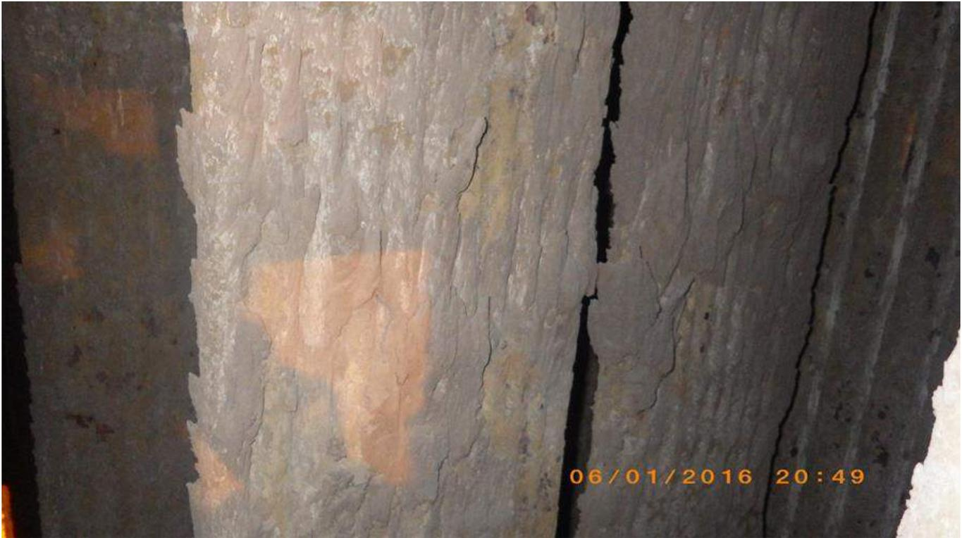
Photo 8 - Second Pass Superheater Platen – Expected Fouling
