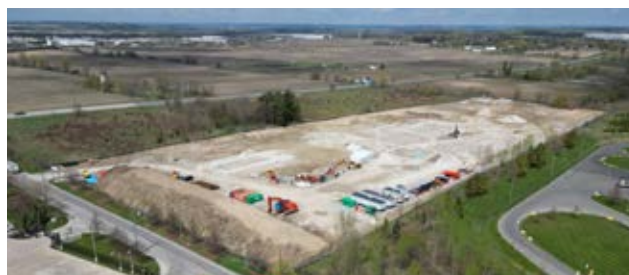
Convertus Biofuel Facility under construction
